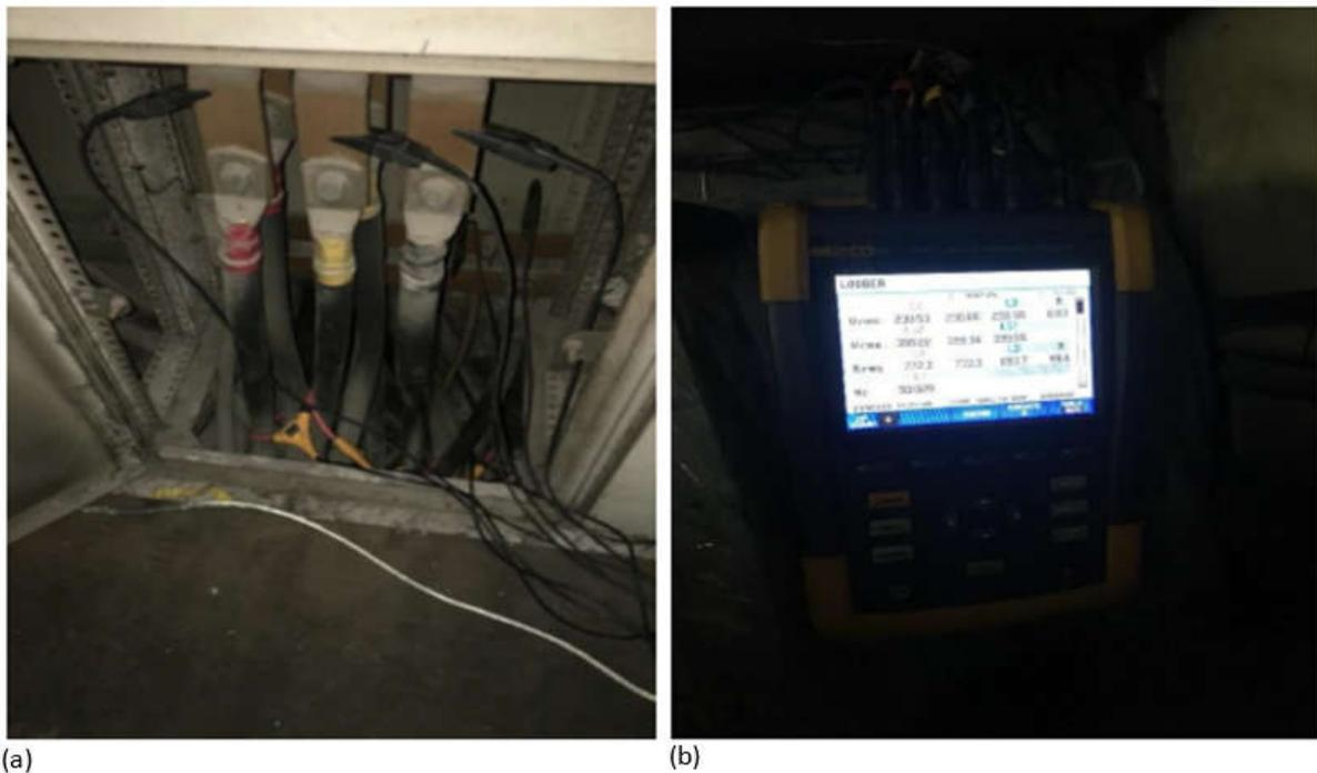
Fig. 3 (a) Installation of Fluke 435 Series II power quality (b) Measurements from installed Fluke 435 Series II power quality analyser at one of the load points [7].
